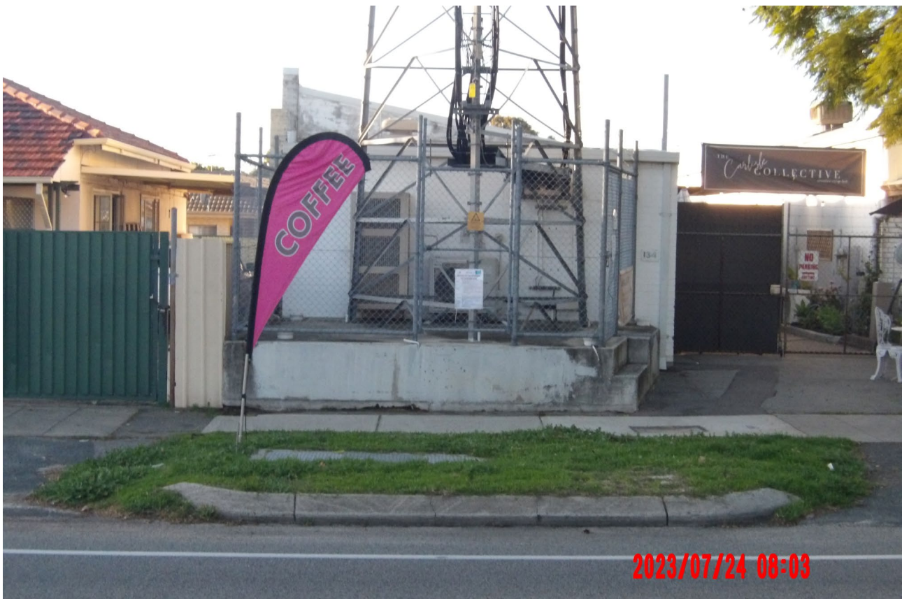
Figure 7: Ground view of existing access arrangements. Upgrades to the foundation are proposed.
