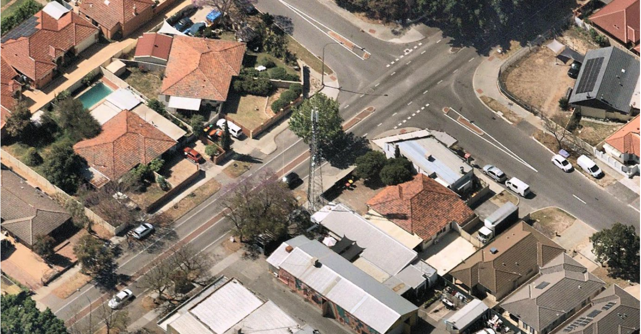
Figure 4: Oblique view of existing facility facing north (Nearmap, October 2022).
