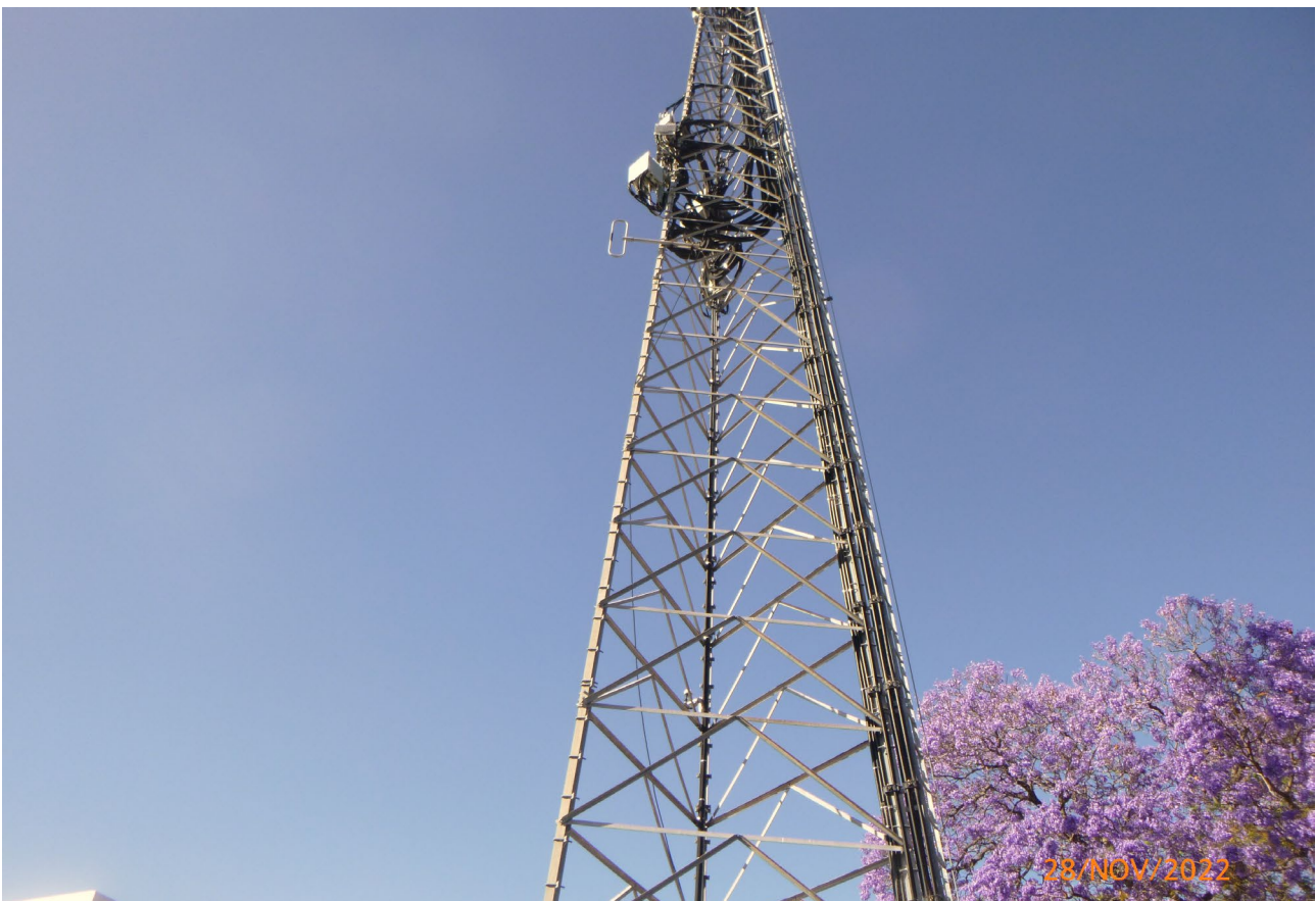
Figure 1: Existing lattice tower to be removed following proposed monopole installation
