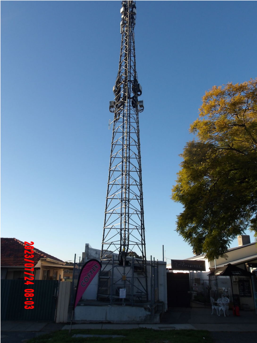
Figure 6: Ground view of existing facility facing south-east
